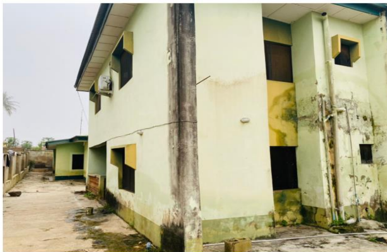
Plate 7. Plumbing defect
