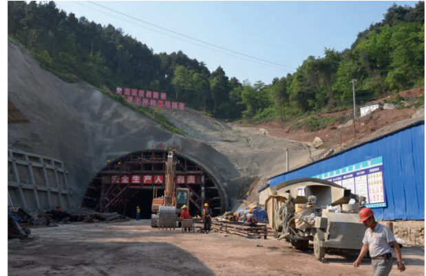
FIGURE 1: Overview of the tunnel.
