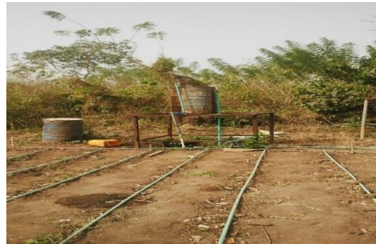
Fig. 2. Installation of low-cost drip irrigation
