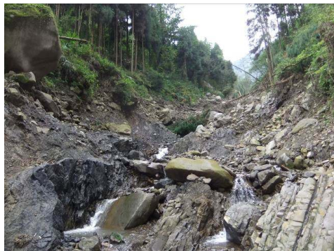
Fig. 7. Washing and erosion in forming region of Xiaowan gully
