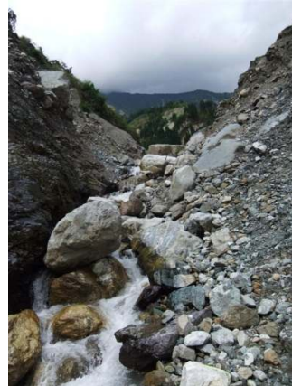
Fig. 10. New water dam in Xiaogan gully
