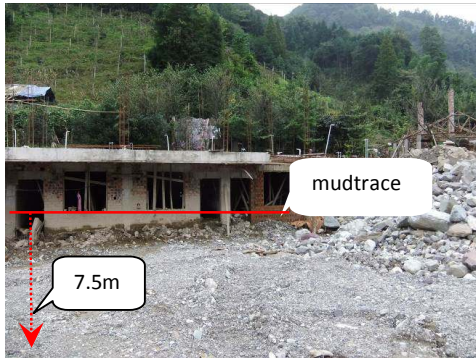
Fig. 5. Houses was destroyed and silted in Jianjianshu
