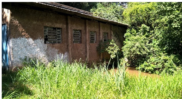
Figure 8. Garcia's PGH façade
